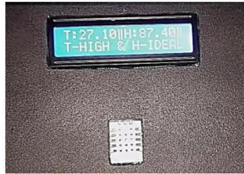
Figure 18. Output Monitoring System (LCD)
