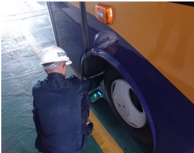
Fig. 14.. Image of sensor installation on the machine
